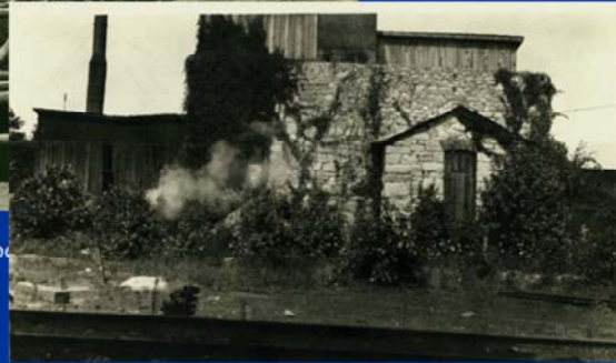
Boiler/Fan House for the Grove Shaft
