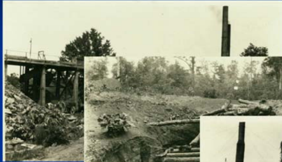
Boiler house, overhead track
