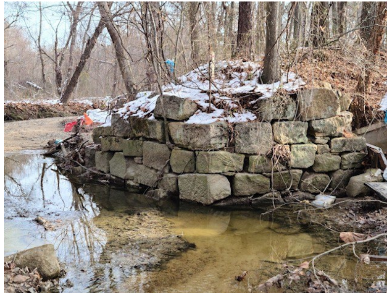
Photograph 34. An abutment for the New York and Richmond Railroad from Hungary Station to Springfield Mine. Courtesy of Rob Timmins.
