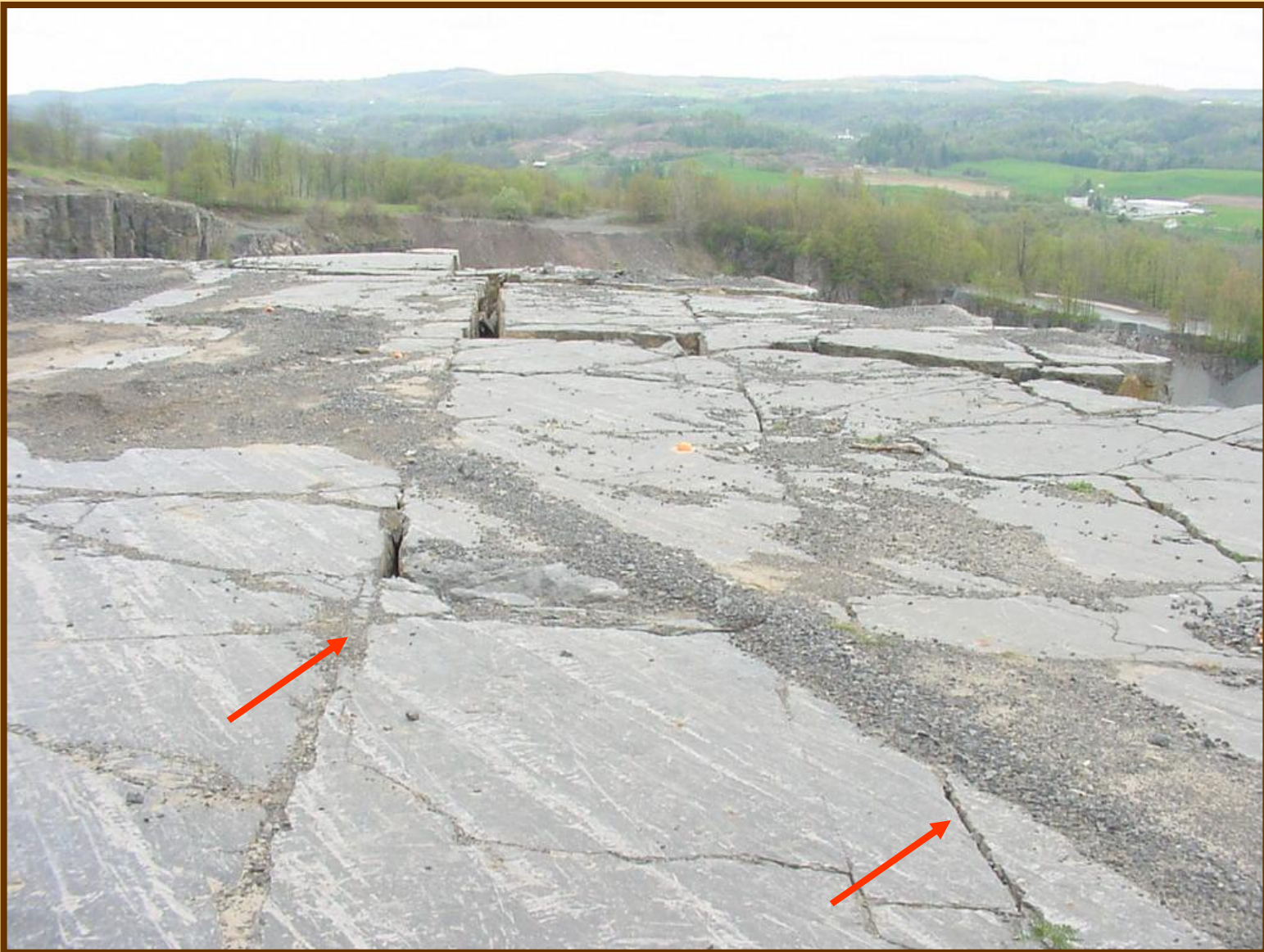
Joints Relative to the Highwall Face
