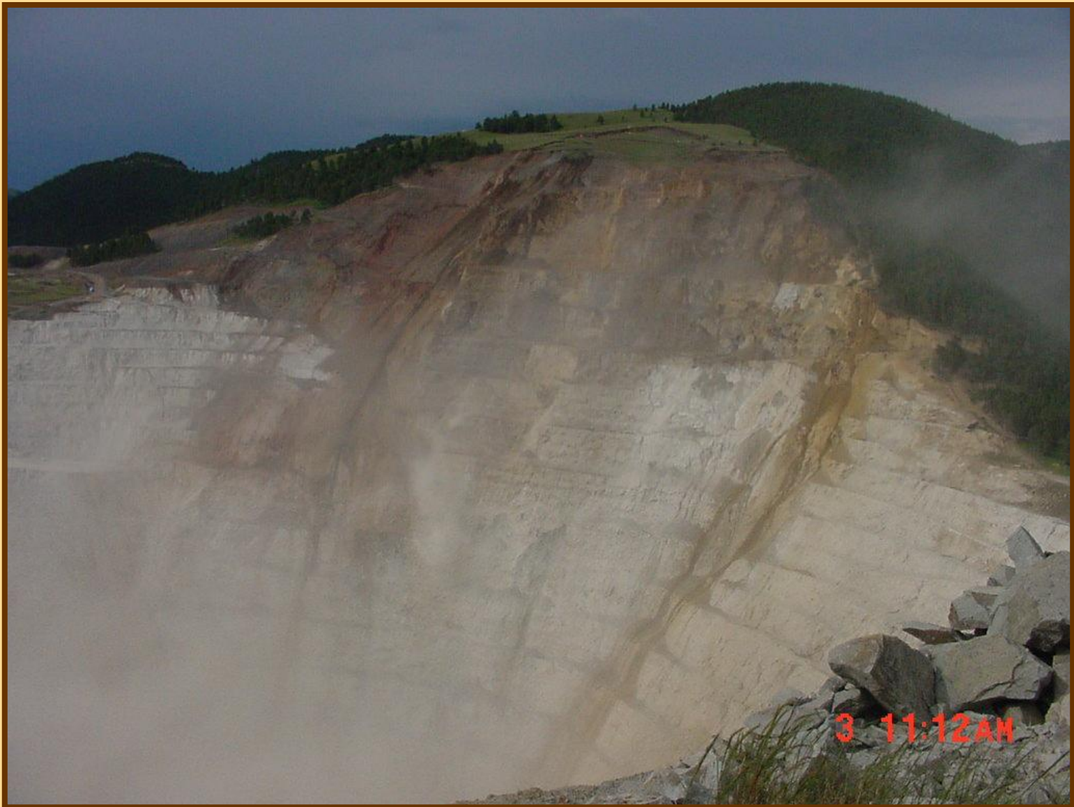
Circular Failure - Before
