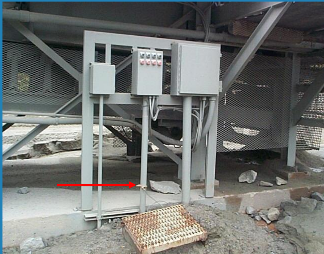
Metal grate bonded to metal conduit
