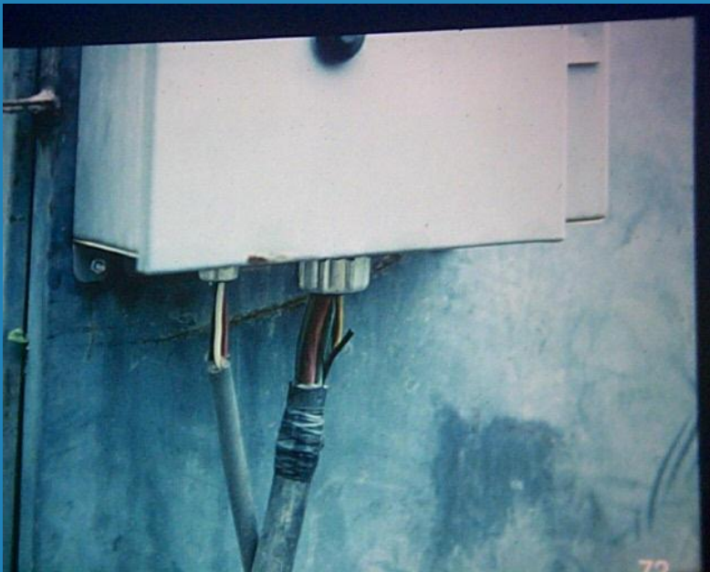
Defective insulating bushing
