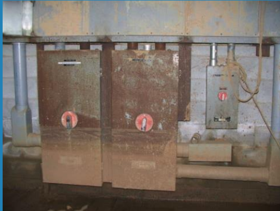
Water damaged equipment & wiring.
