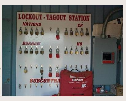
➤ Shut off, lock and tag any circuits or machinery in close proximity that might pose a hazard too!
