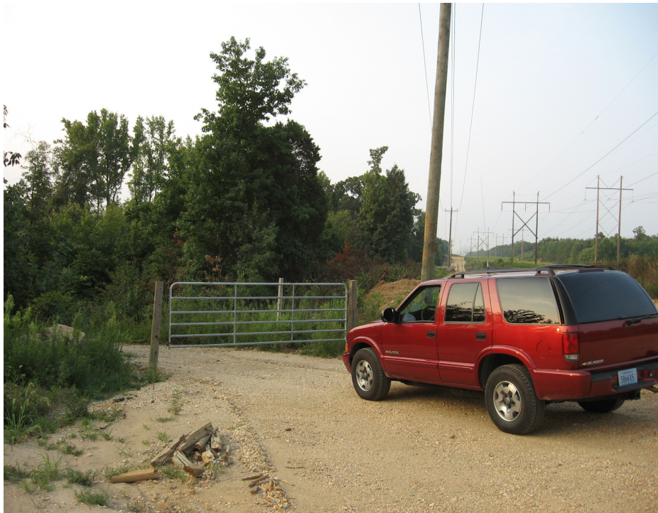
Locked gate, but no warning sign as required.
