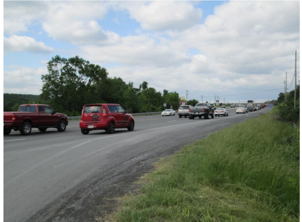
Busy highway impacted by recent flyrock incident
