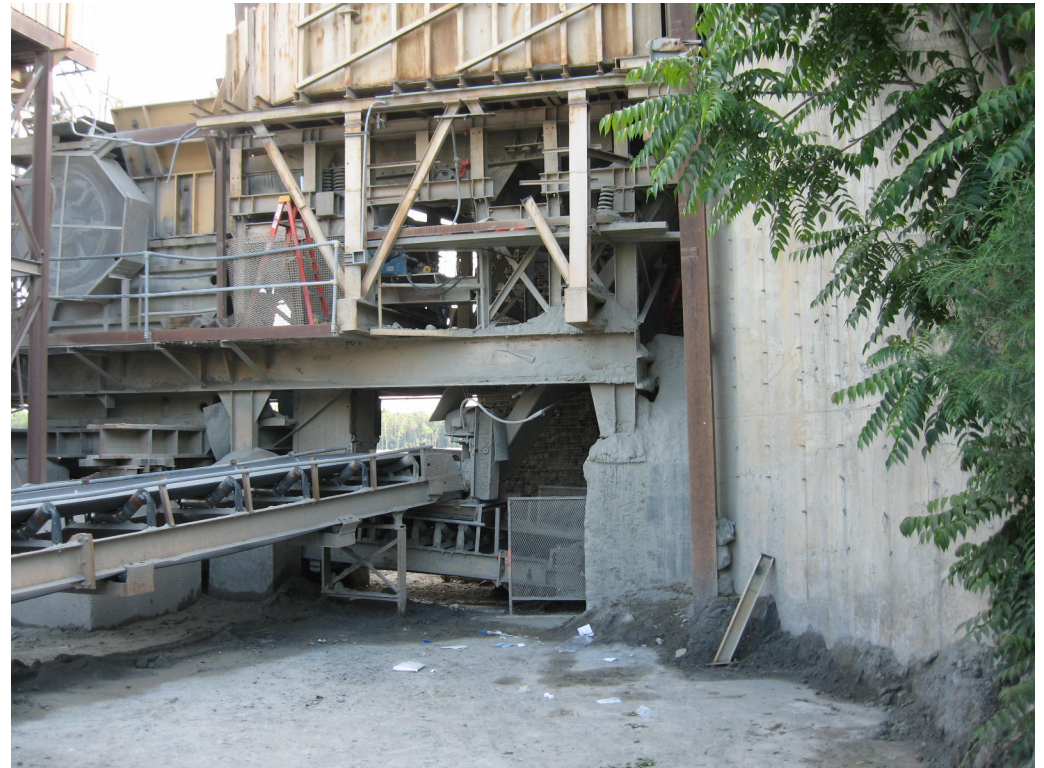
Miner fell from platform at top center of photograph
