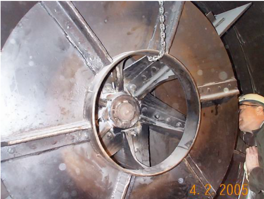
Exhaust fan that was being installed.
