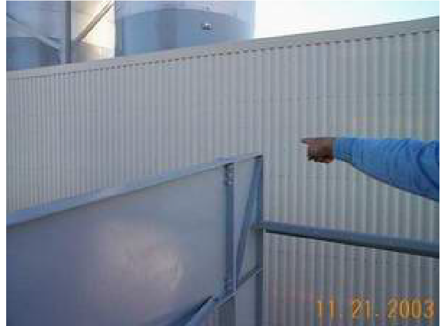
Close-up photo showing location where miner was sitting before he fell.
