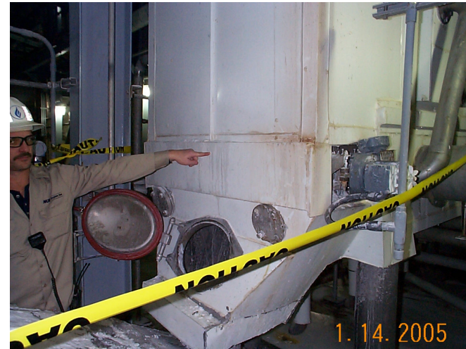
Approximate location of rotary valve inside dryer
