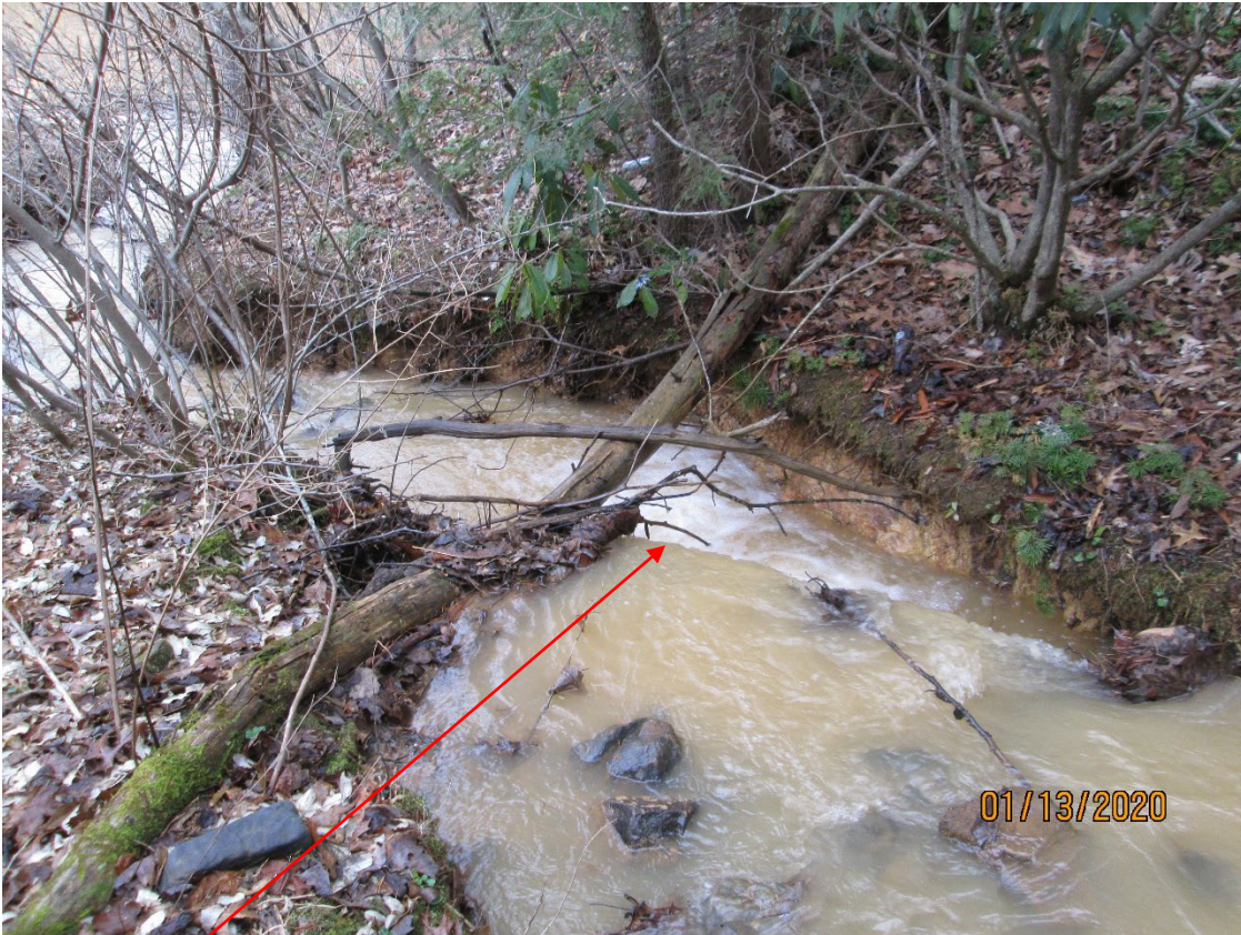
Edge of existing drainage channel. Channel was blocked, so water overflowed and washed out a new path.
