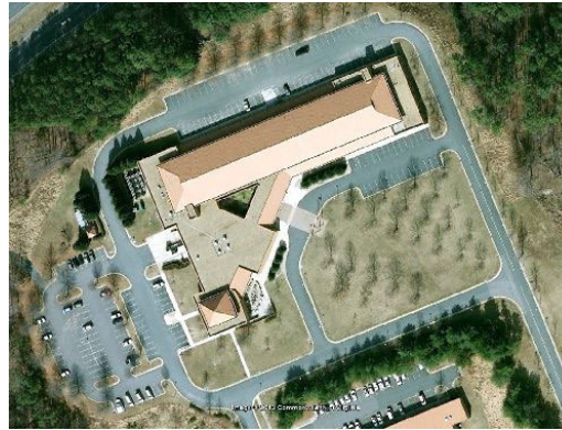
Geology and Mineral Resources Program Main Office
