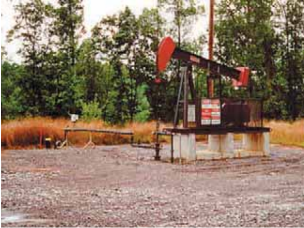
Figure 47. Pump jack installation on coalbed methane well operated by CNX Gas Company, LLC, in Buchanan County. Photograph provided by the Division of Gas and Oil.
