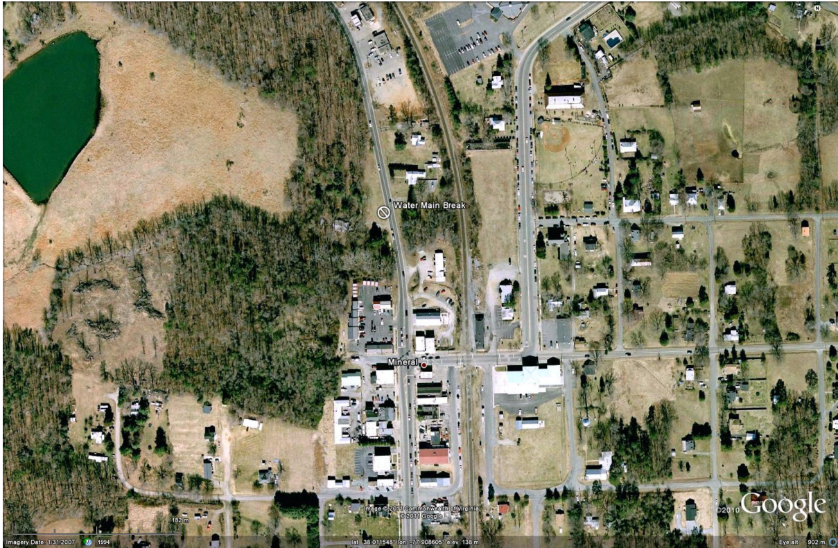
Figure 21. Aerial image of Mineral showing the location of the water main that broke during the earthquake.
