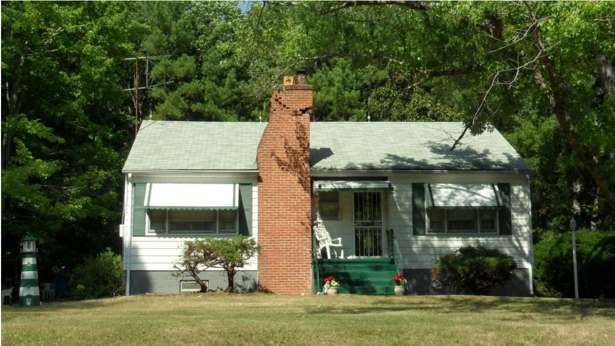
Figure 52. Typical damage to brick chimneys (37.9966, -77.9631).
