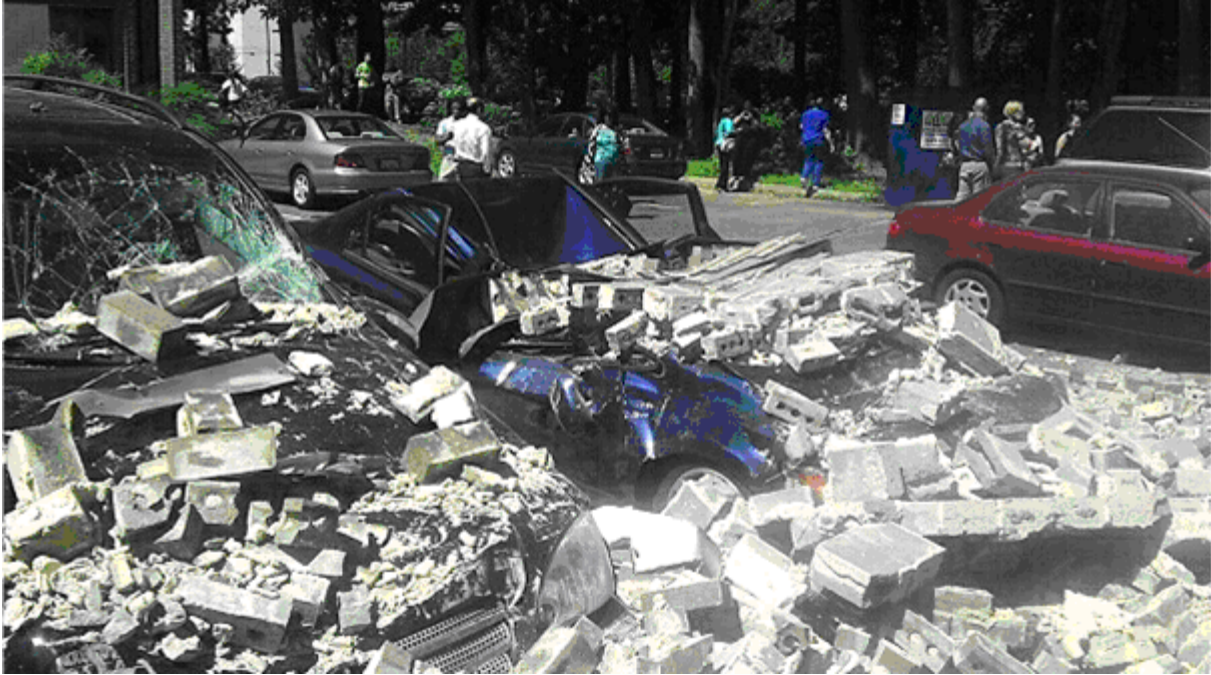
Photo: damage from unreinforced masonry wall collapse in the Washington DC area.
