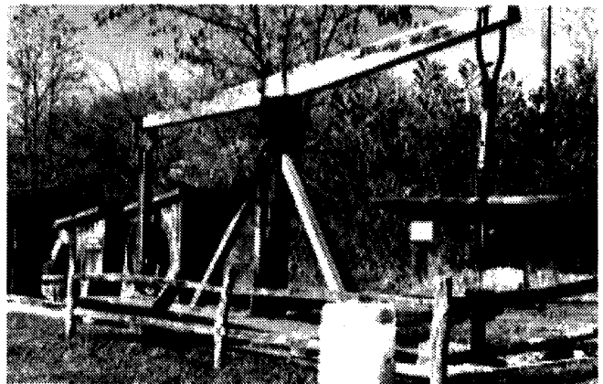
Figure 7. Salt Park on south side of Saltville with shed and furnaces and walking beam brine pump.
