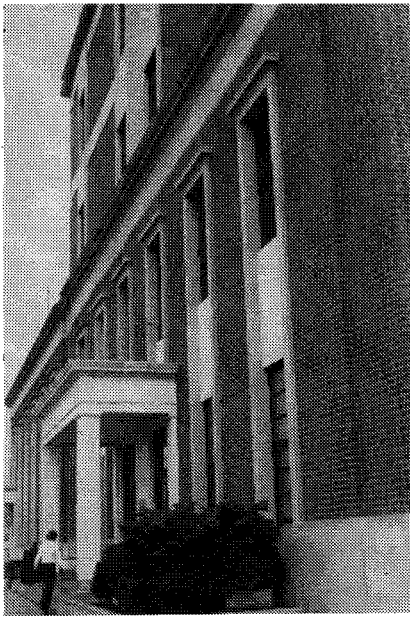
Figure 24 Centel building, City of Charlottesville
