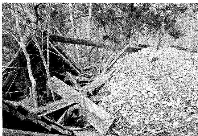
Figure 4. Collapsed headframe at northernmost shaft, High Hill mine.
