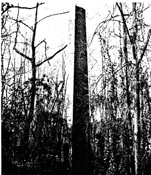
Figure 2. Brick roasting stack at the Grasty mine tract, Orange County.
