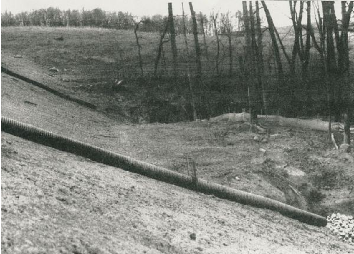
FIGURE 8. Example of temporary slope drain
