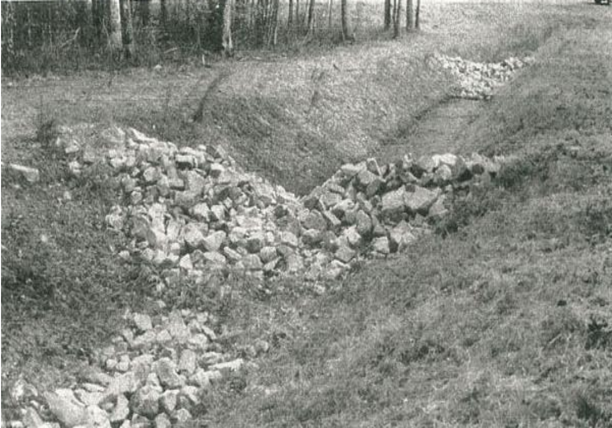
FIGURE 2. Example of a rock check dam
