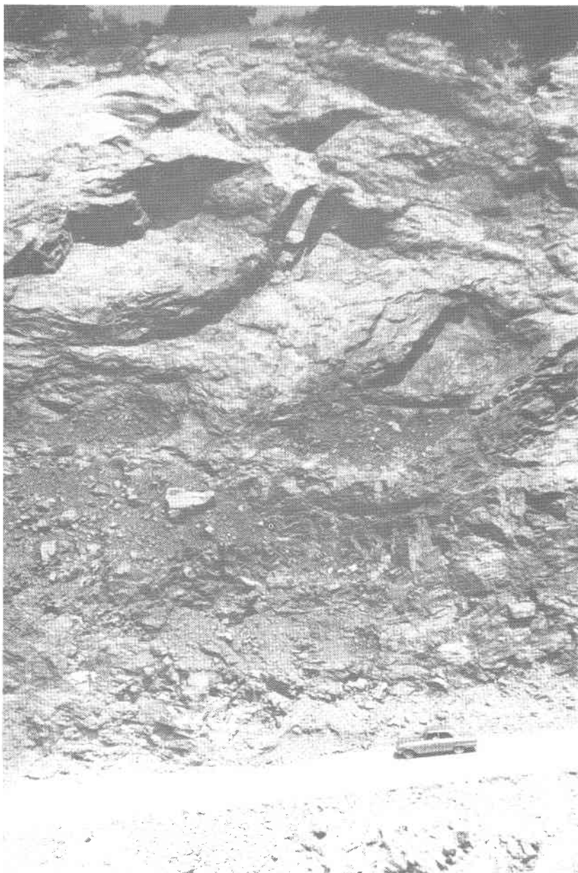
Figure 22. Vulcan Materials Company quarry (Plate 1, No. 11); contorted, steeply dipping Chepultepec limestone is thrust over gently inclined Lenoir-Mosheim Limestone. Fault trace is located in photograph about 0.25 inches above automobile.
