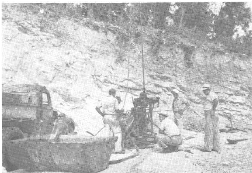
B. Exploratory diamond drilling at the Coles mine, Bedford County (1947).
