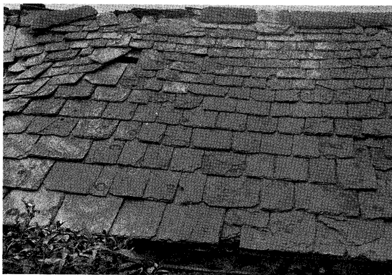
B. Loudoun slate on an old building near Turnbull, Fauquier County. The roof has not been repaired since the close of the War between the States.
