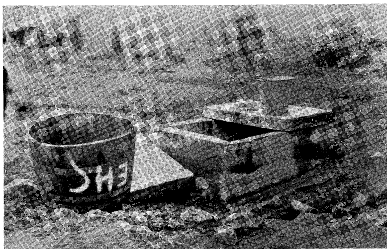
B. An unsanitary spring. Surface drainage enters the spring through openings beneath the improperly set concrete spring box.
