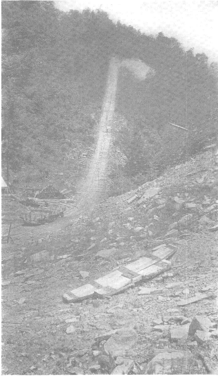
(A) Incline at Matoaka No. 2 mine.
