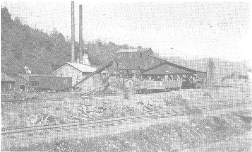
(A) Slope and tipples of Big Vein Pocahontas No. 2 mine near Pocahontas.
